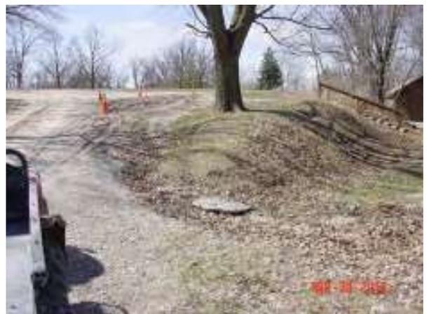
The catch basins, which were previously created, need to be uncovered and protected from damage. The drainage pipeline from those basins needs to be routed to avoid damage and the ditches need to be improved to avoid further erosion. Additionally, the wooded area to the north of the parking lot should be cleaned up a storm water detention area may be created to minimize down stream damage from runoff.
