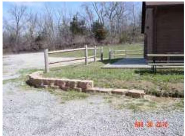
The project area is northwest of the trading post. Last year the Landscape Architecture merit badge class worked on a project that was constructing a CMU (concrete masonry unit) seating wall. The project progressed well but was never completed. The wall needs to be completed three blocks high. This will provide accessible seating to individuals who are not wheelchair bound.
