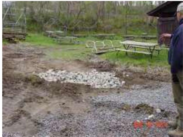
**6. Drainage repairs to gullies developing in the turf banks of the new shooting sports area.**
